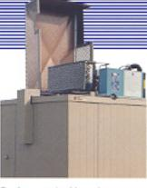
Roof mounted refrigeration system — Completely assembled, wired and test run at the factory. Easy access for service.
